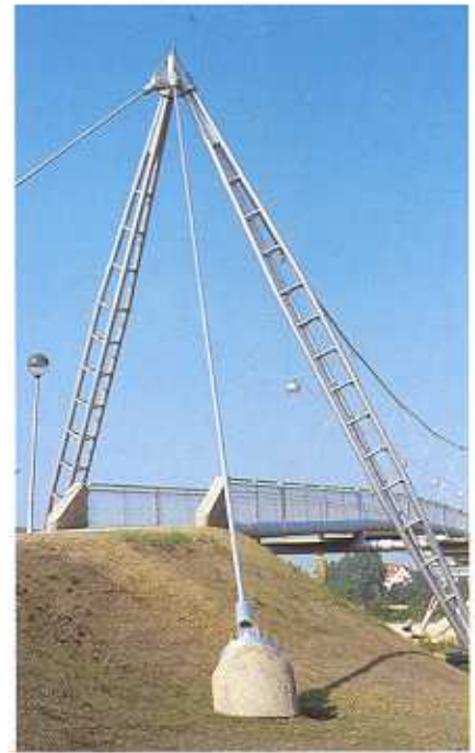
Footbridge at Munich
